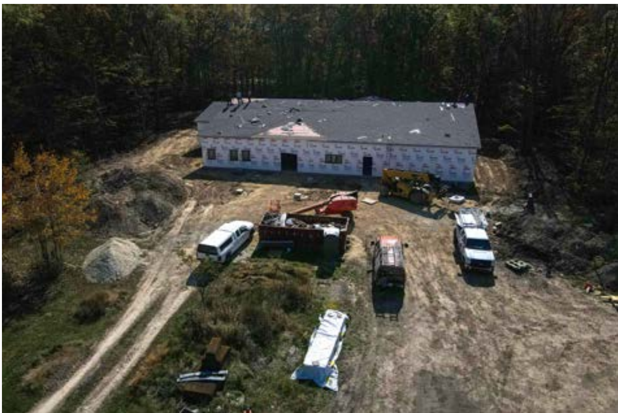
Progress on the new CREO community building. Photo by Doug Peconge.
