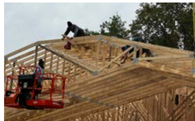
Trusses being set. Photo by Doug Peconge, CREO.
